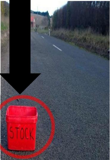
Facing the wrong way & puts the truck over-taking the site in danger. No control in place.
